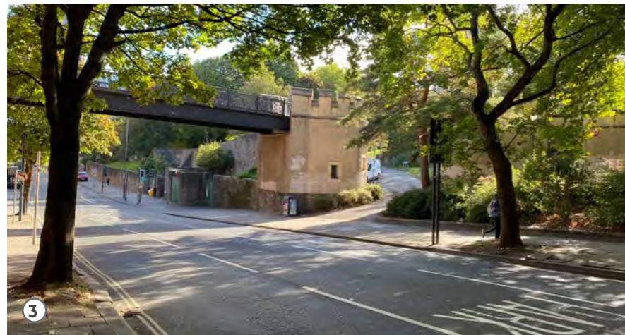
1. View from Union Street across Newgate into Castle Park 2. View along Newgate towards Broadweir 3. View along Newgate to the bridge to the Galleries
