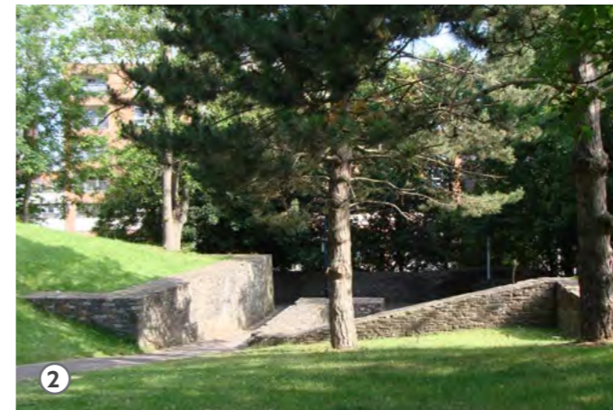
Fig. 94 Existing walls within Castle Park
